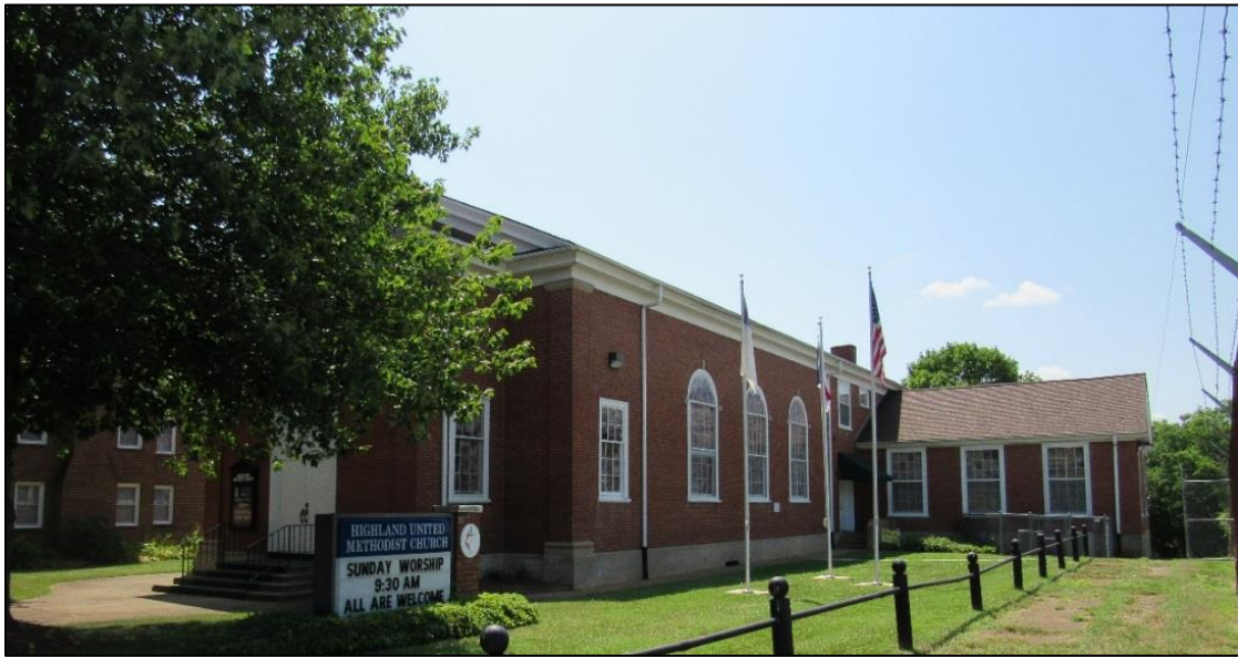
Photo 8: Highland Methodist Church (GF8602), Northwest Oblique.
