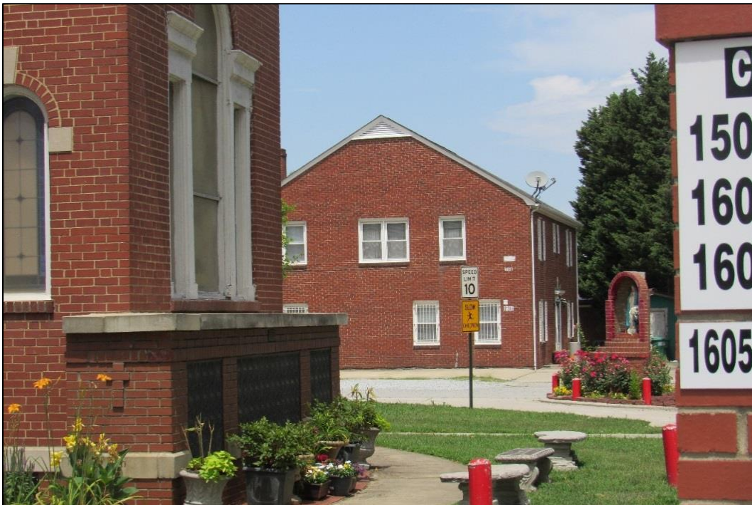
Photo 6: Christ the King Catholic Church Educational Building (GF0448), Looking Northeast.
