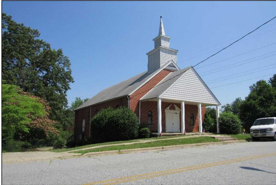
Photo 3: Highland Baptist Church (GF8689), Southwest Oblique.
