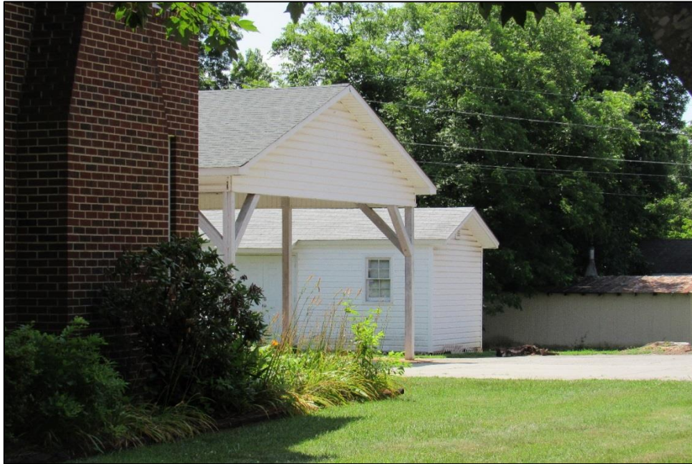
Photo 10: Highland Methodist Church Parsonage (GF8601), Shed and Carport, Looking Southeast.
