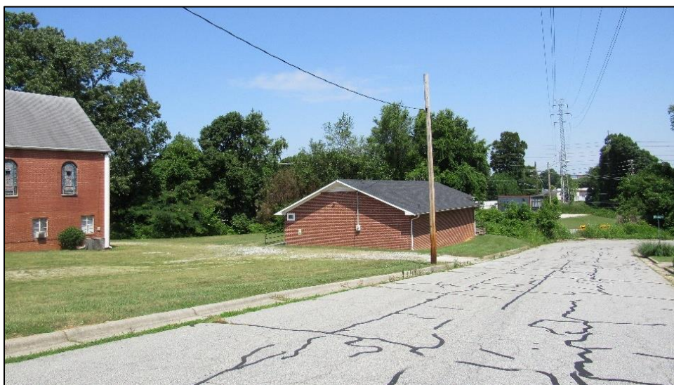
Photo 4: Fellowship Hall at Highland Baptist Church (GF8689), Southeast Oblique.
