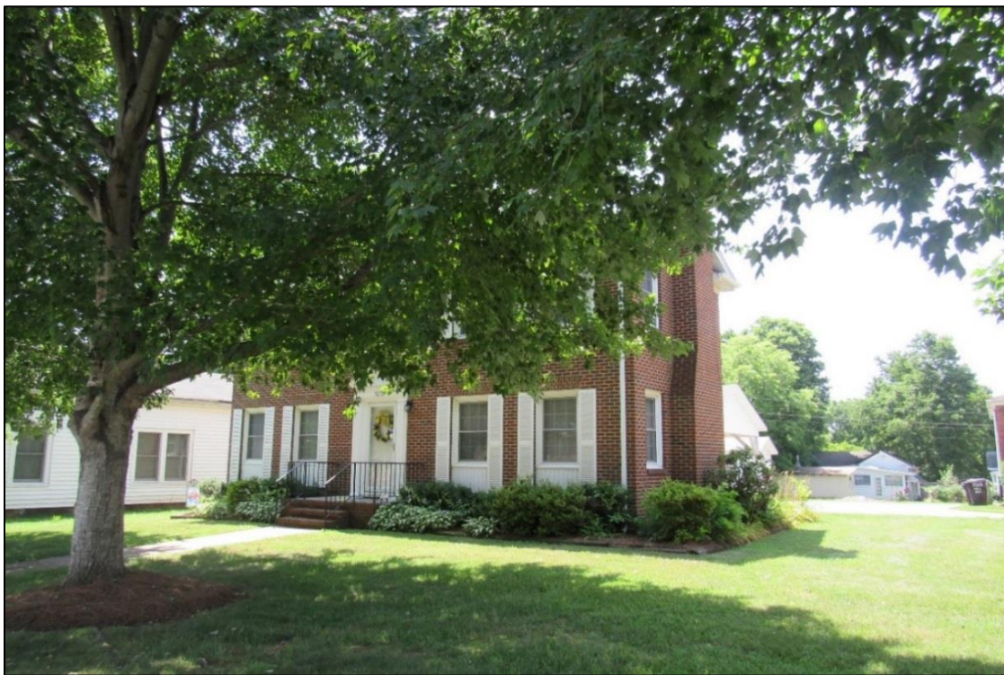
Photo 9: Highland Methodist Church Parsonage (GF8601), Northwest Oblique.
