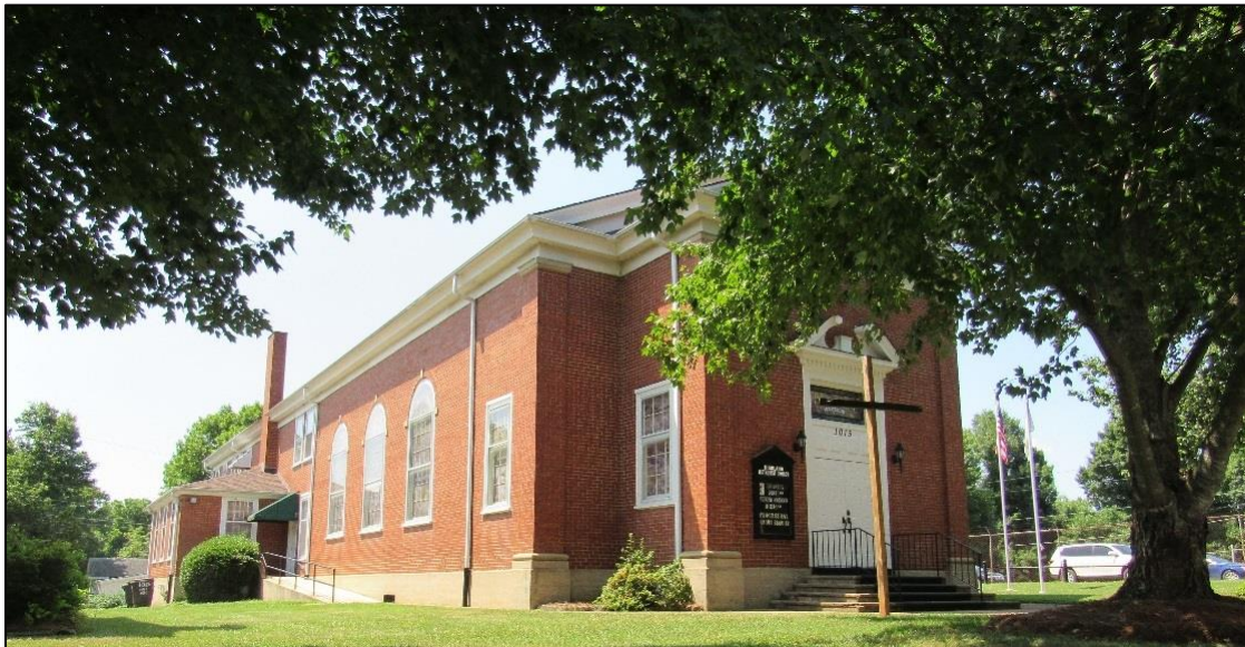
Photo 7: Highland Methodist Church (GF8602), Northeast Oblique.
